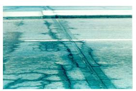
However, it is the vehicular traffic on the road which is the major cause of road deterioration, especially on heavily trafficked roads. Every vehicle which passes over a road causes a momentary, very small, but significant deformation of the road pavement structure. The passage of many vehicles has a cumulative effect which gradually leads to permanent deformation and road surface deterioration by cracking.
